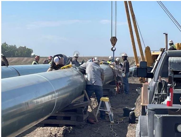
Facing south at MP 33.9, K&K welding mainline pipe
