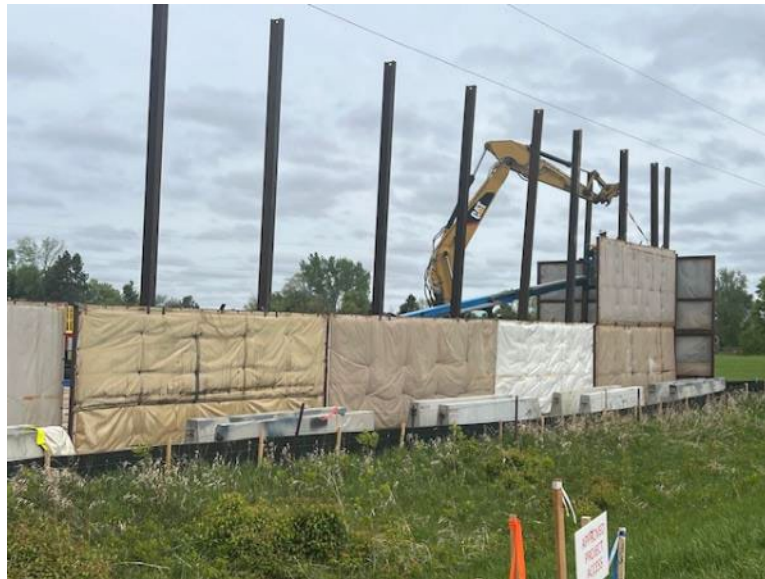
Facing north on HDD P4-3, sound wall installation ongoing
