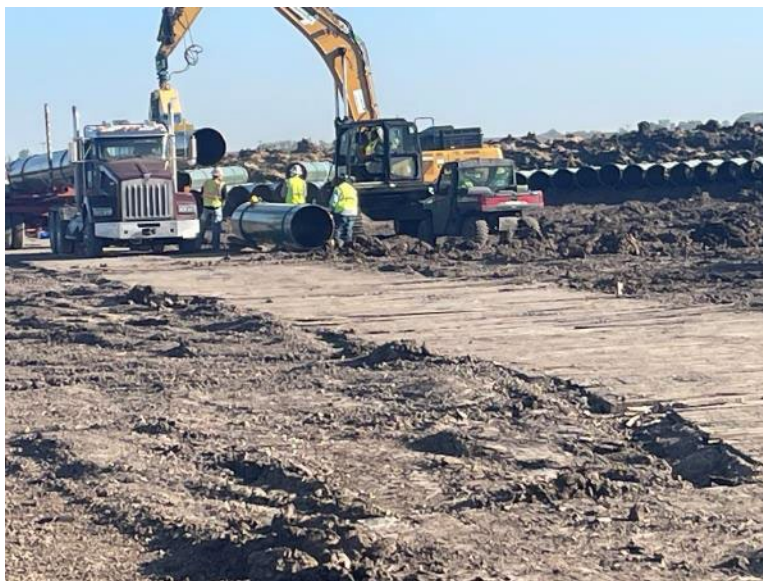
Facing north at MP 34.2, contractor unloading line pipe
