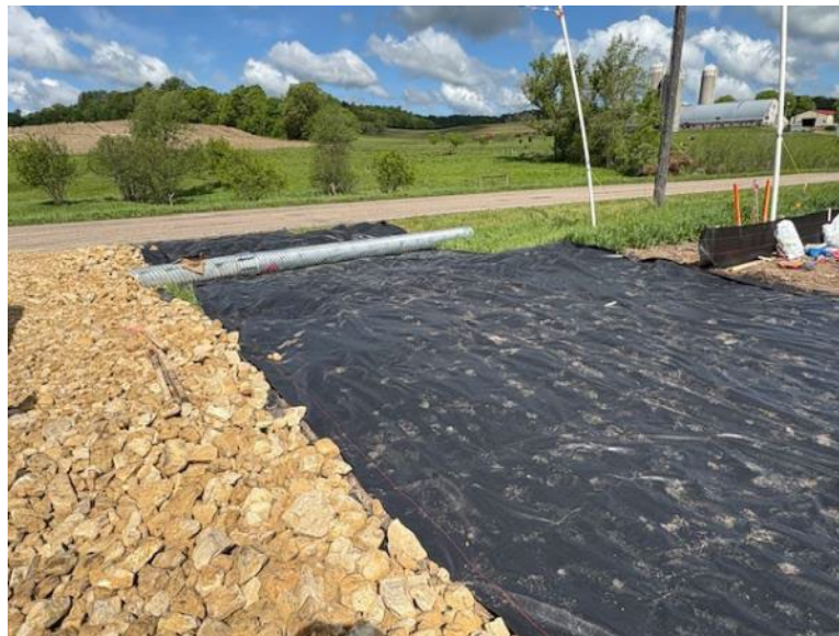
Facing northwest near MP 3.5, contractor installing geotechnical fabric and flume pipe
