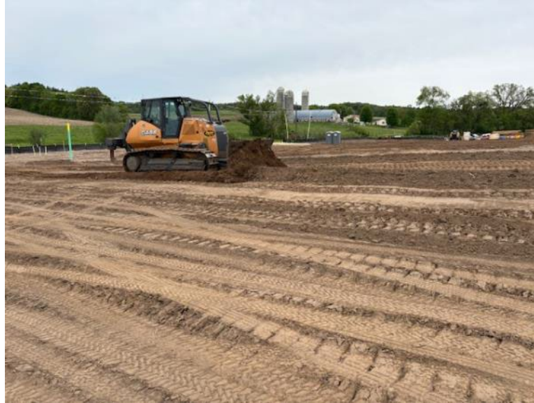
Facing north near MP 3.5, contractor stripping topsoil
