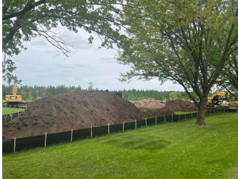
Facing north near MP 2.3, topsoil segregation ongoing
