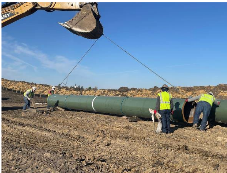
Facing southwest at MP 33.8, K&K stringing mainline pipe
