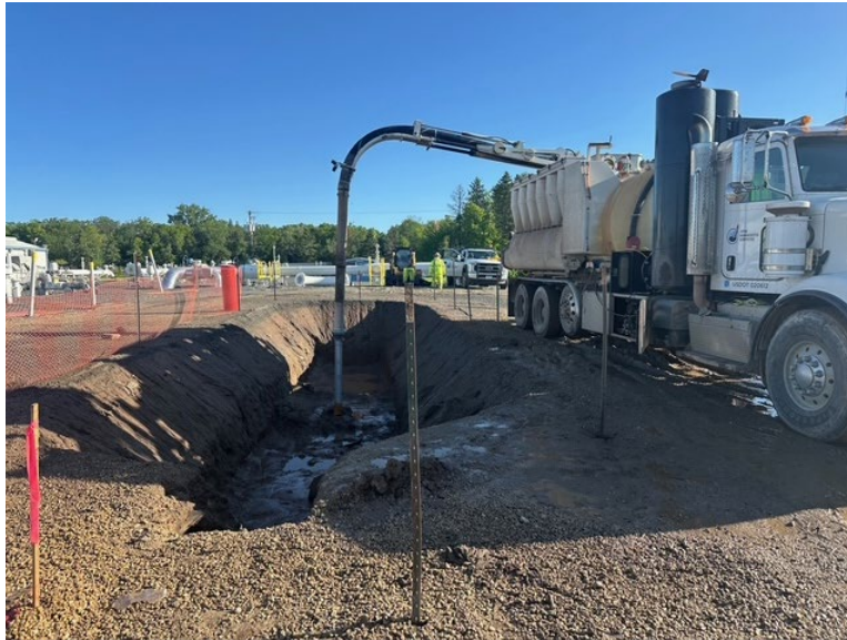
Facing north in the Hugo compressor station, contractor performing hydro-vacuum excavation
